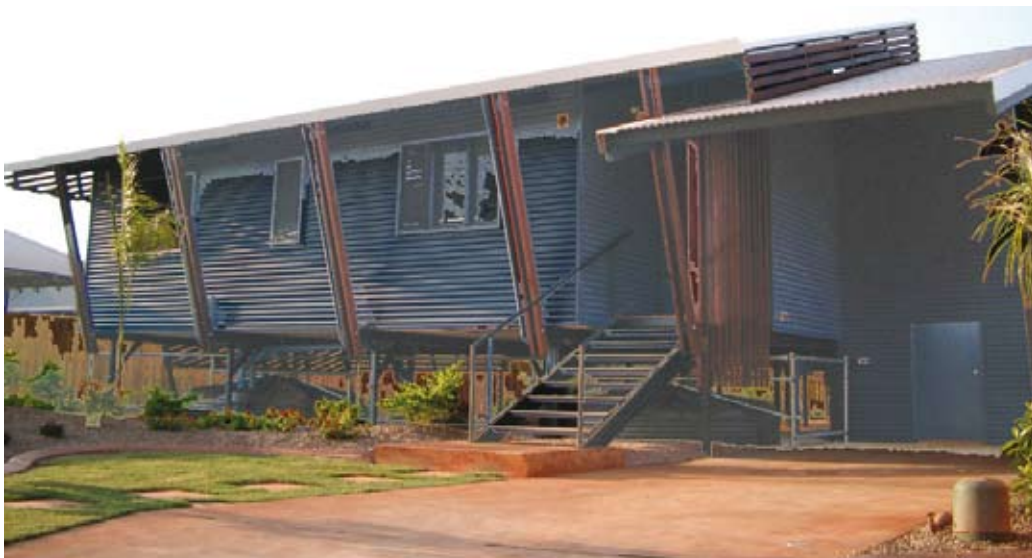
Figure 1. Broome 'Filter House'
