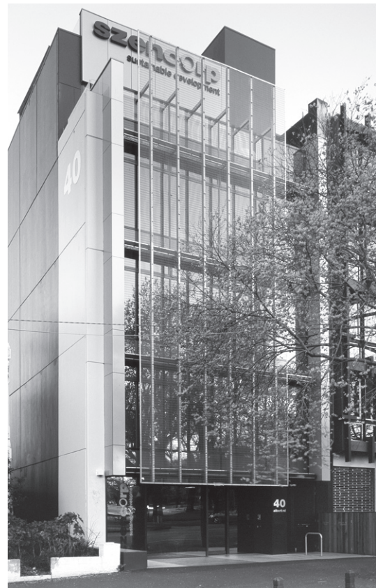
Figure 1. Albert Street Facade
