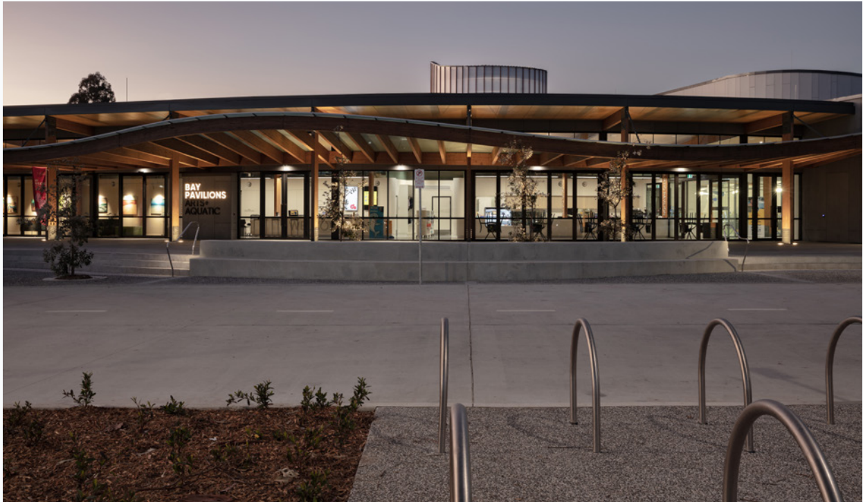
Figure 16. The main entry from the western forecourt is defined with an undulating awning element that includes specially fabricated double curvature glue laminated beams. (Image: Alexander Mayes Photography)
