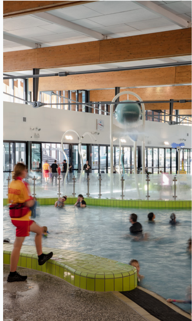
Figure 9. The aquatic pool hall features hybrid glulam and steel bowstring trusses. The trusses support R6.1 high performance sandwich panel roofing and high-performance double glazing to reduce heat loss, while the northern orientation facilitates passive heat gain through the cooler months. (Image: Alexander Mayes Photography)
