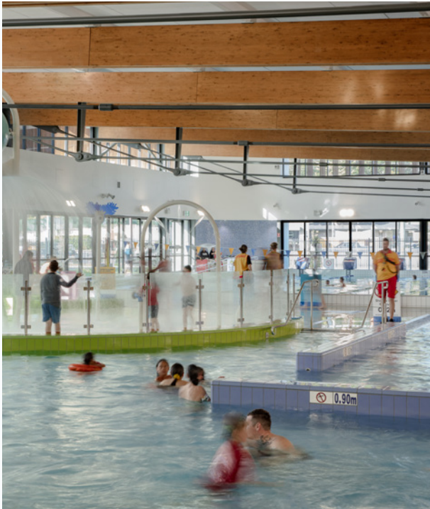
Figure 7. The indoor aquatic hall features a number of different water bodies that cater to a wide range of activities including lap swimming, aqua-aerobics, learn to swim, recreation and warm water therapy. Pool filtration utilises UFF technology that substantially reduces water usage over conventional pool filtration. (Image: Alexander Mayes Photography)
