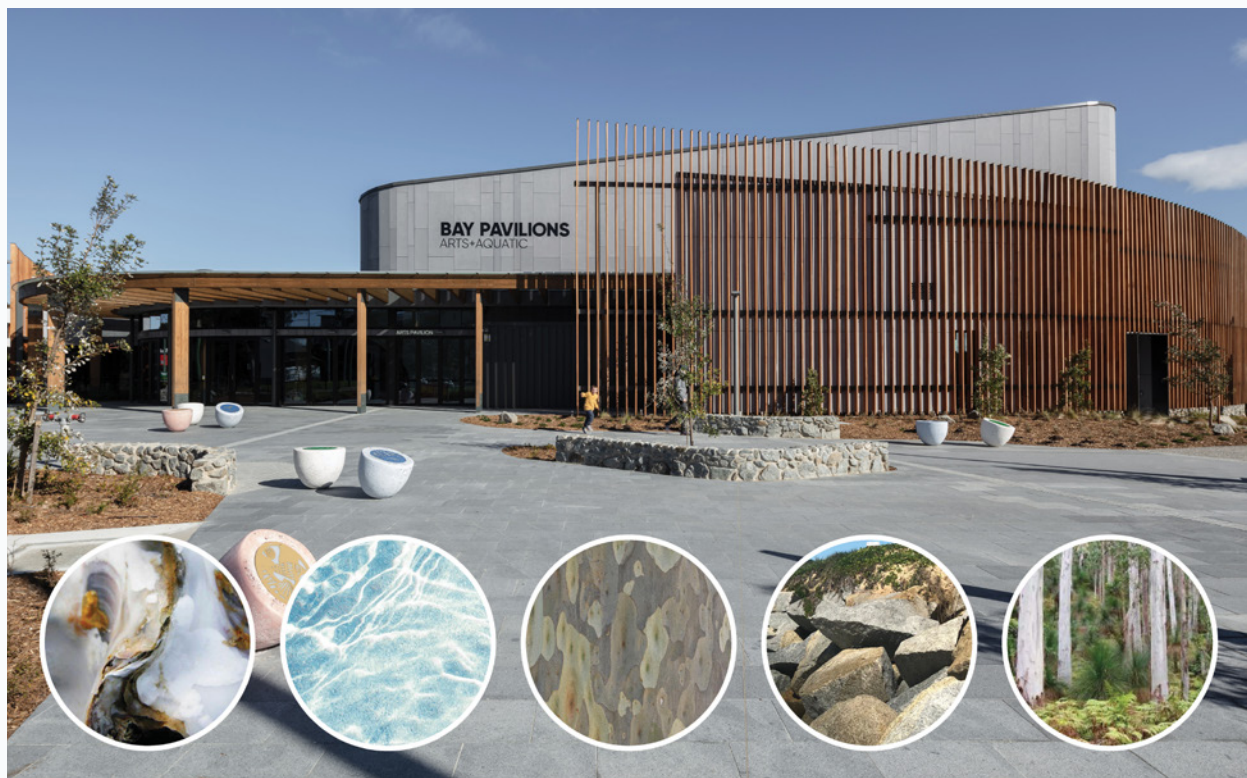
Figure 4. Facade materiality and expression responds to the strong connection between people and place. The project utilised locally sourced materials including granite from Beashel Quarries and sustainably sourced hardwood for the external timber screens. (Image: Alexander Mayes Photography)
