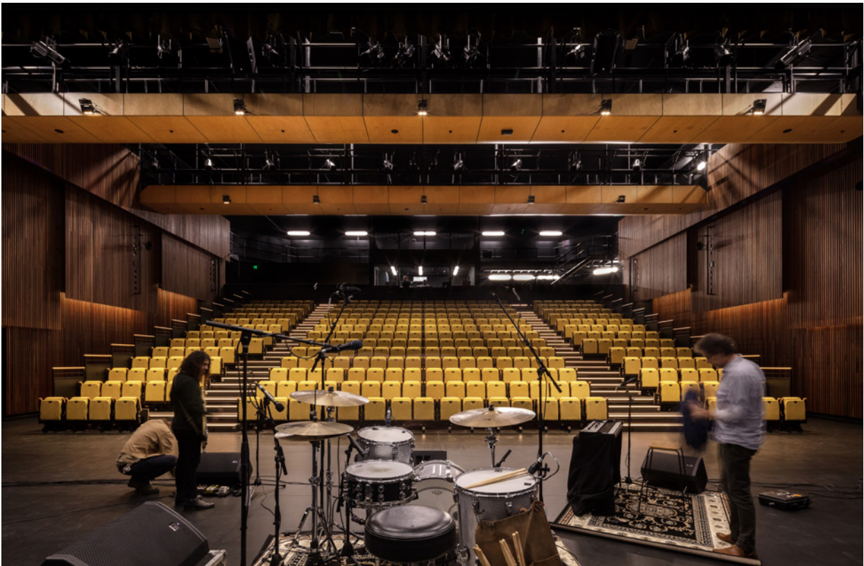
Figure 8. The Whitlams setting up for a gig in the Theatre on the opening weekend. The Theatre makes extensive use of spotted gum timber battens and hoop pine ceilings for acoustic attenuation. (Image: Alexander Mayes Photography)
