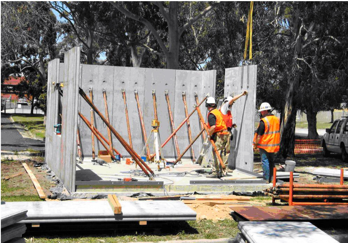
Figure 1 Precast LBCM panels being lifted and propped in test house at, CSIRO Highett, Melbourne
