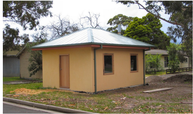
Figure 6 The completed test house at CSIRO Highett, Melbourne
