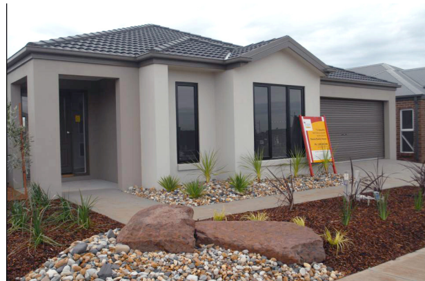
Figure 7 Precast LBCM panel house, Werribee, Victoria
