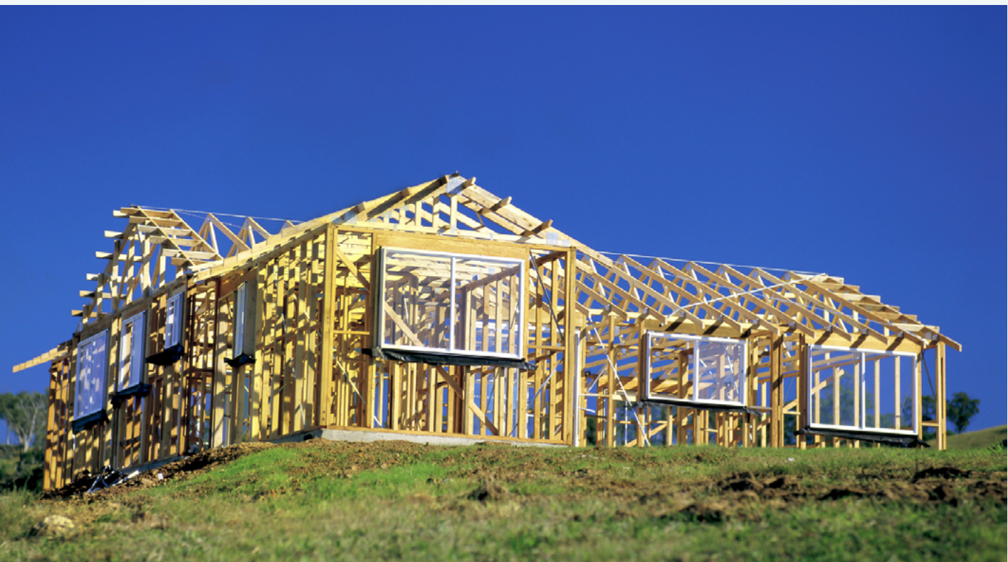
Figure 1: House under construction, Sydney (Image: iStock)
