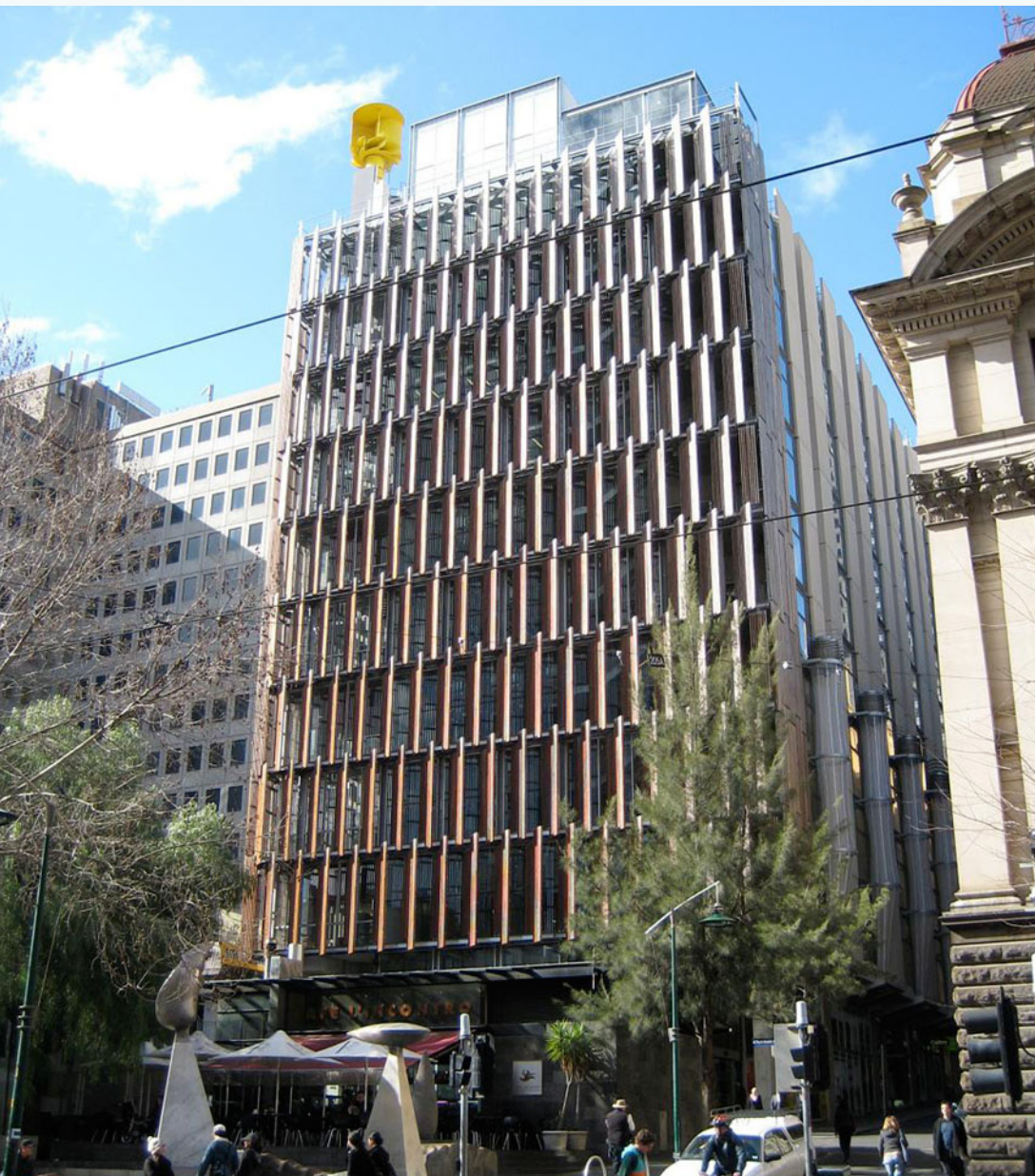
Figure 1: Melbourne's Council House 2 (CH2), a 6-star Green Star rated building with a post-occupancy evaluation to back up its design rating.
