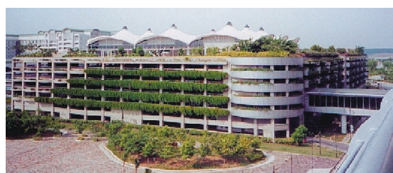
Figure 6. Kuala Lumpur airport (courtesy of Ronstan International, 2002)
