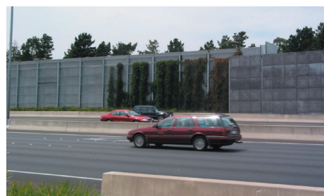
Figure 7. Freeway noise attenuation wall (courtesy of Transurban 2002)
