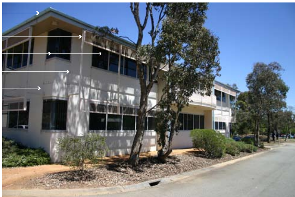
Figure 1. Existing building exterior (Source: Kevin Miller)
