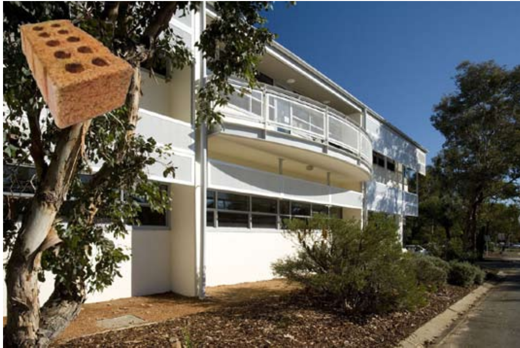
Figure 3. Thermal mass was captured (Source: Kevin Miller)
