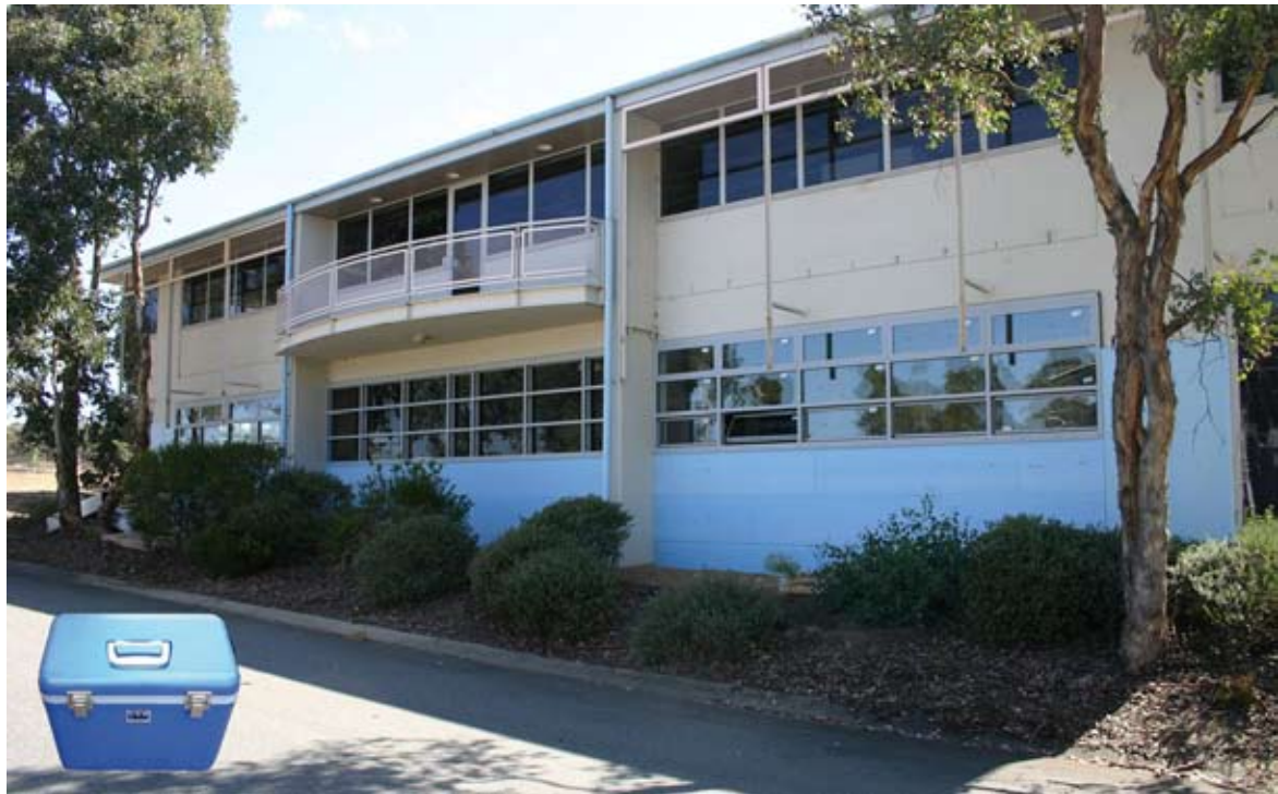
Figure 2. Thermal insulation was added
