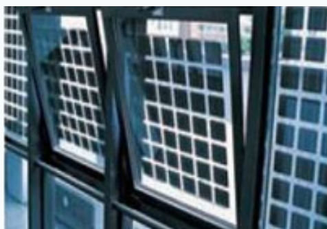
Figure 6: Monocrystalline glazing modules at Daito University, Itabashi Campus, Tokyo
