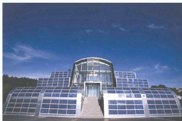
Figure 8: 22kW PV System, Institute for Marketing, Upper Austria
