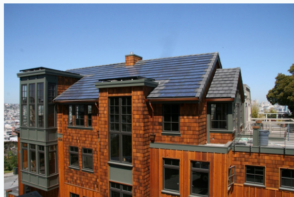
Figure 14: Century Roof and Solar Installation, California (Image: Suntech)
