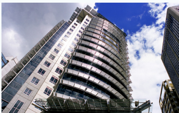
Figure 13: Brisbane's William Buck Centre, designed by Hassell Architects, has an innovative BIPV solution with grid-connected solar awnings (Image: Hassell Architects / David Sanderson)
