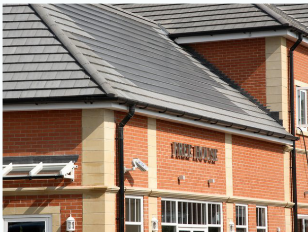
Figure 23: Heritage building retrofit with Solar Century C21e Roof Tile, UK (Image: Solar Century)
