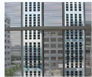
Figure 21: Translucent PV modules at Daito University, Itabashi Campus, Tokyo (Images: Ben Nakamura / Yamamoto Hori Architects)
