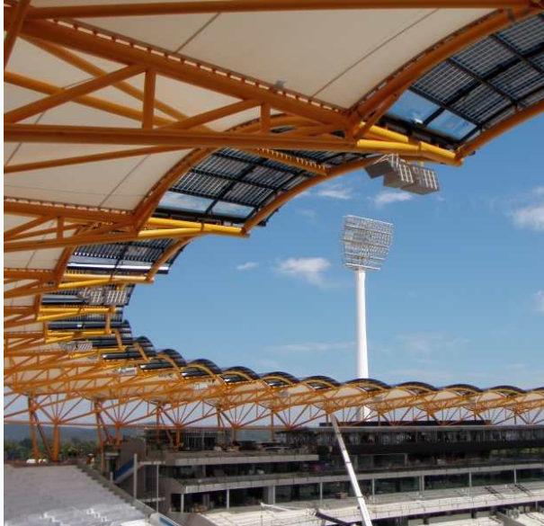
Figure 19b: PV awnings, Gold Coast Stadium, Qld (Image: Stoew Engineering)
