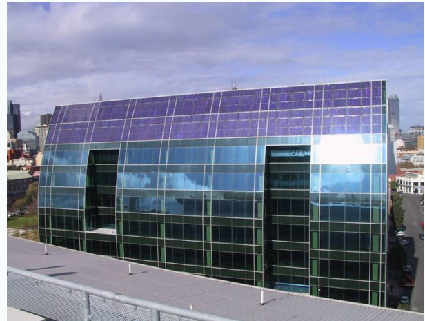
Figure 10: 43kWp PV glazing façade, Melbourne University, Australia (Source: STI Australia)
