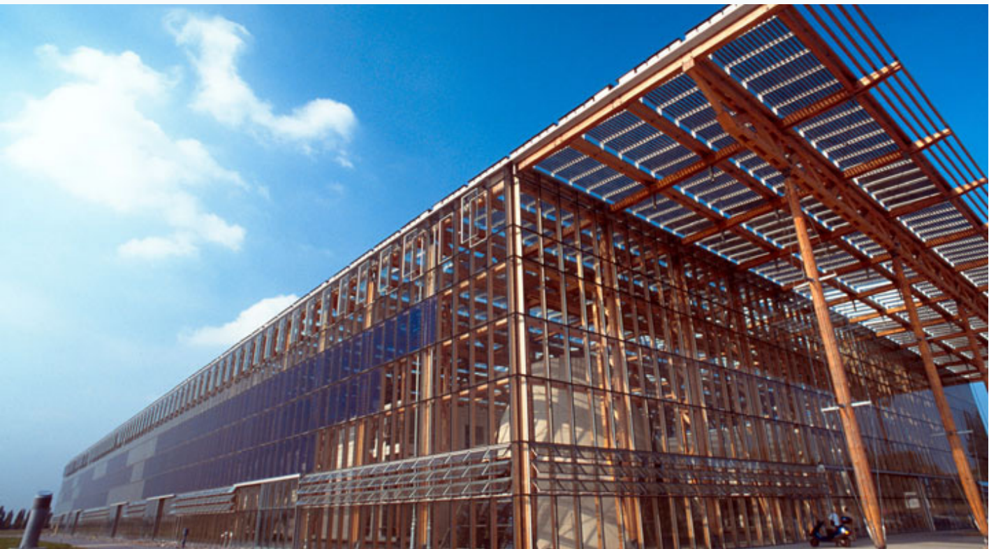
Figure 1: Mont-Cenis Academy building, Herne, Germany. A 1MWp BIPV array (Image: BSW-Solar)
