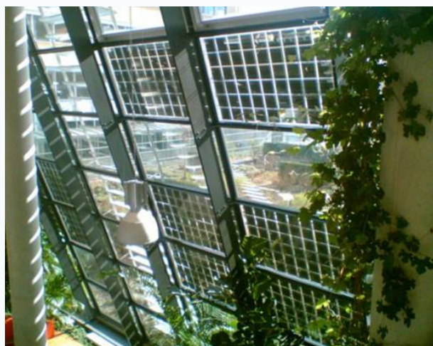
Figure 18: Sloped PV integrated façade, Solar Info Centre GmbH, Freiburg, Germany
