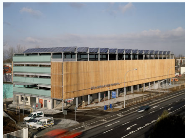
Figure 11: 89kWp Solargarage Vauban, Freiburg. The mounted PV is aligned to the pylons of the building which extend to the ground. (Image: Hotz + Architekten)
