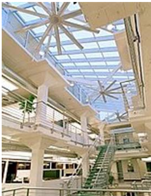
Figure 15. Atria with circulating fans for destratification
