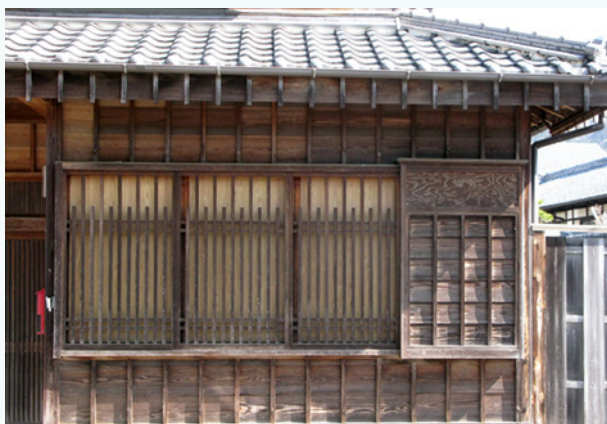
Figure 24: Amado – rain shutters covering the external opening are slid into the box at right
