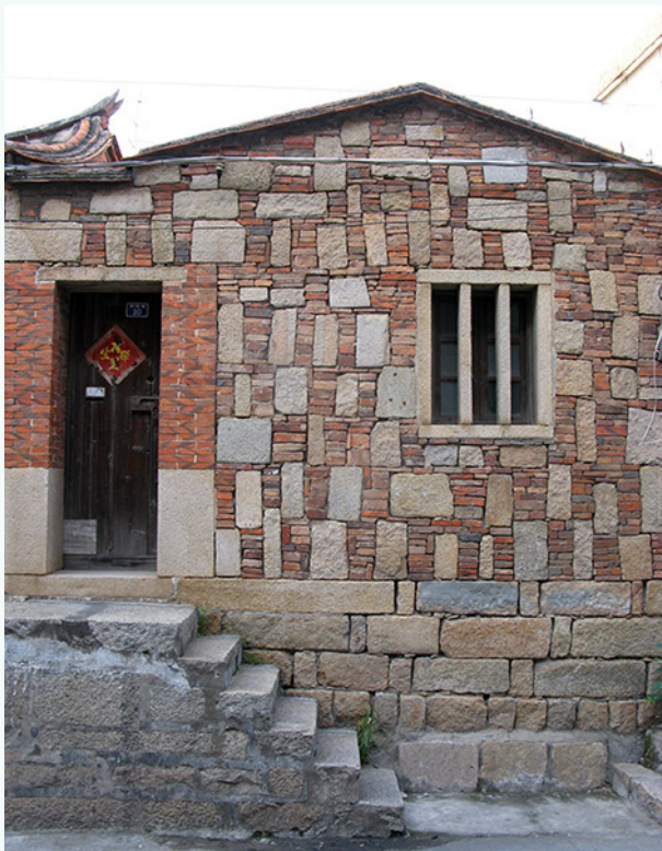
Figure 15: Mixed masonry wall resting on stone base. Fujian
