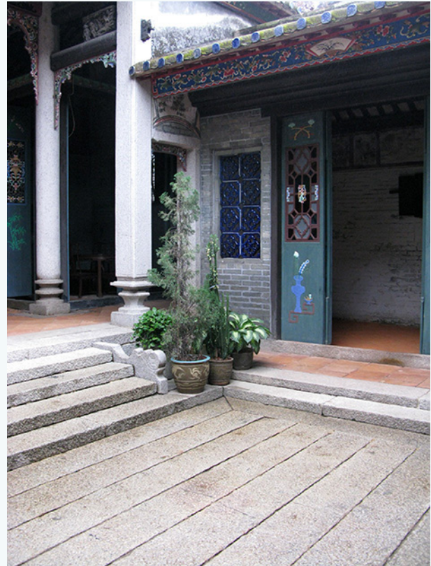
Figure 16: Durable materials used internally and externally, timber columns are lifted off the ground to prevent water damage. Fujian
