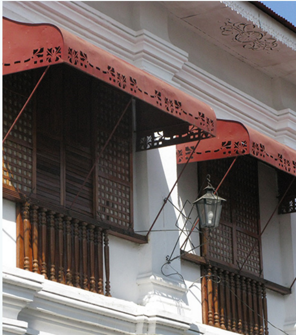
Figure 17: Screens, sunshades and ventilated eaves on a Vigan house
