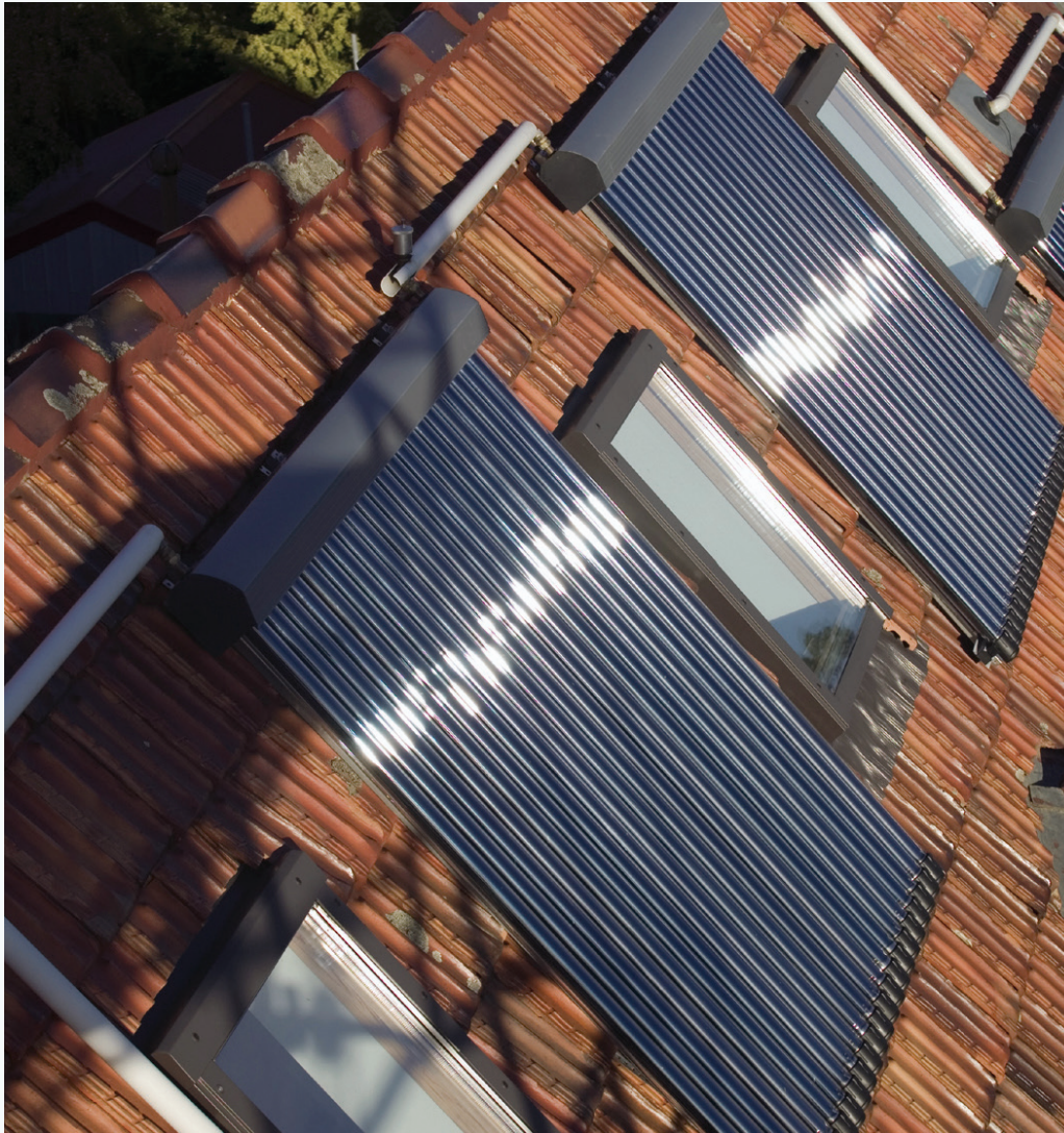
Figure 1. Domestic solar hot water system with evacuated tubes (Image: Alternative Technology Association, 2014)
