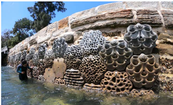
Figure 15. Built structures providing refuge for different species. Living Seawalls. Emulating reef characteristics to provide habitat for marine organisms. (Image: Reef Design Lab)
