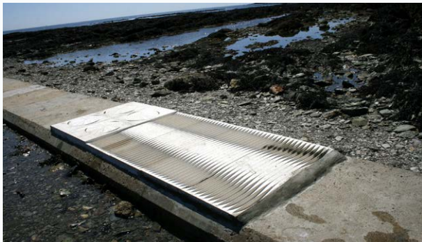
Figure 16. Built structures providing refuge for different species. Walkway tiles for marine organisms. (Image: Daniel Metcalfe)
