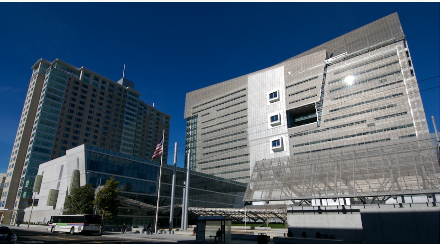
Figure 1: Thom Mayne's San Francisco Federal Building (Wikimedia Commons)
