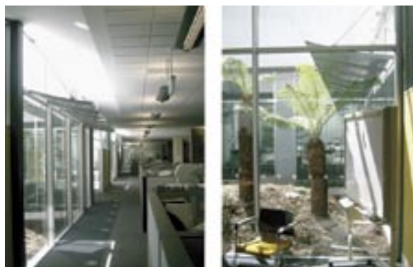
Figure 4. Internal and external views of light shelves from courtyard
