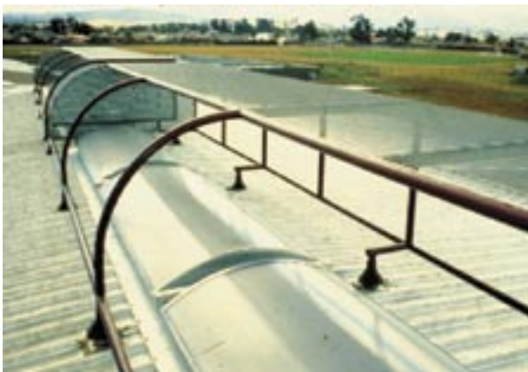
Figure 6. External view of skylight with steel mesh shading
