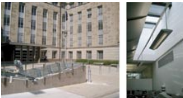
Figure 2. External and internal views of skylight penetrations
