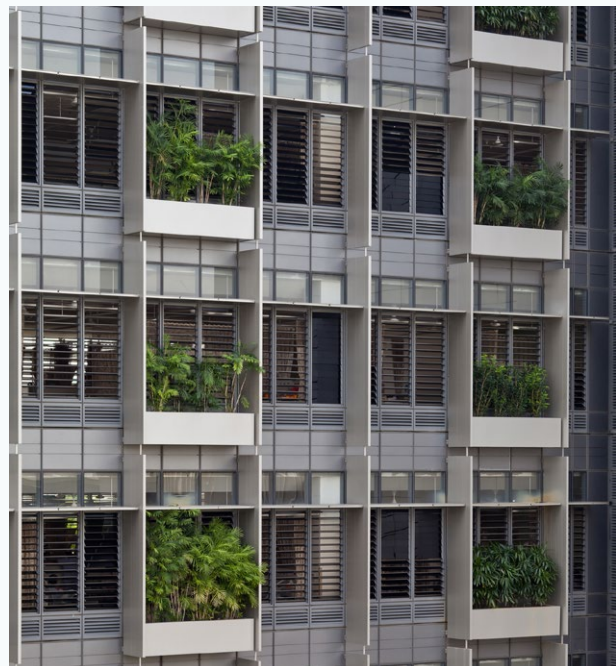
Figure 11. Khoo Teck Puat Hospital by RMJM and CPG Consultants (Architect of Record). Air flows up the building, carrying the scent of plants to hospital beds (Image: RMJM)
