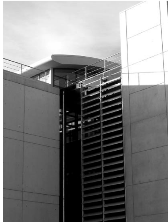
Figure 3. North view of the lift shaft and louvres to the west end of Building T (source: Deakin University)
