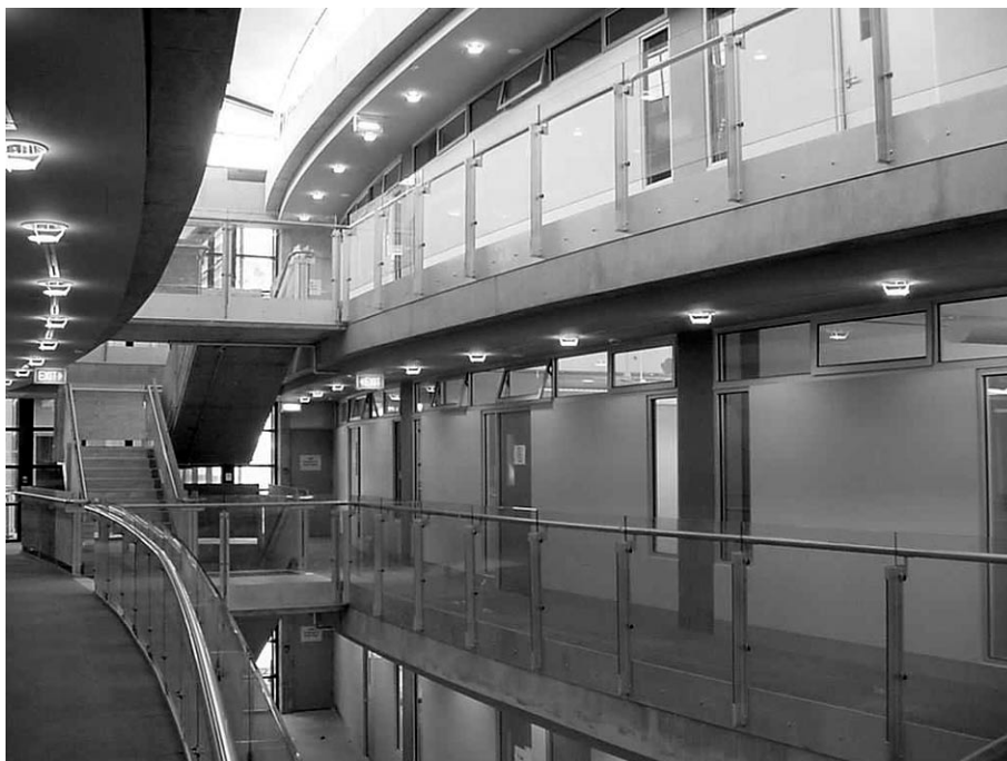
Figure 2. Interior of Building T (source: Deakin University)
