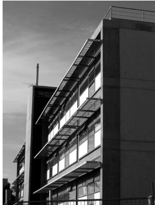
Figure 7. The north facade of Building T (source: Deakin University)
