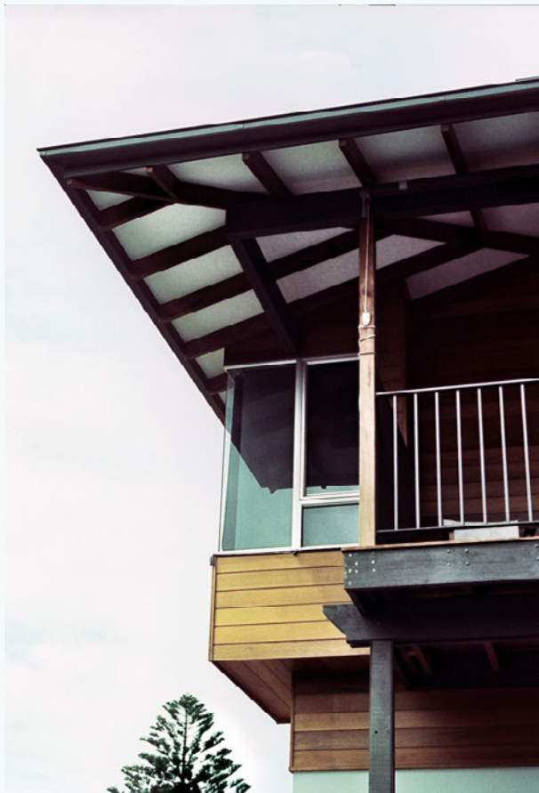
Figure 5: Extended overhangs for effective sun shading
