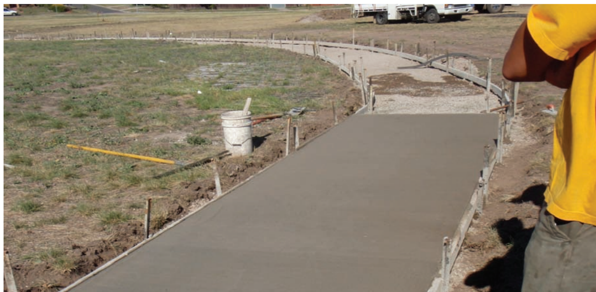
Figure 1. Concrete with geopolymer binder being used in footpath construction in Hume City Council, Victoria
