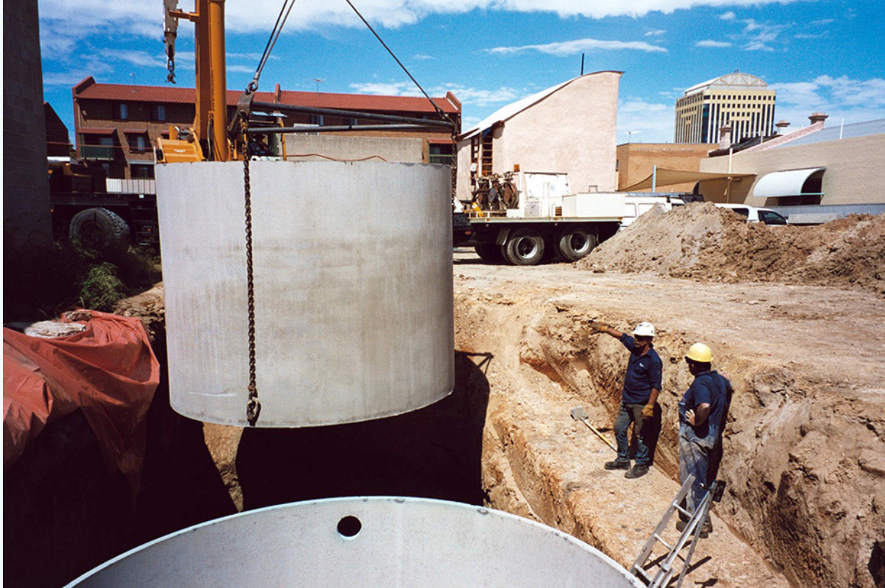
Figure 10: The two 20,000L underground tanks being installed beneath the carports at Christie Walk
