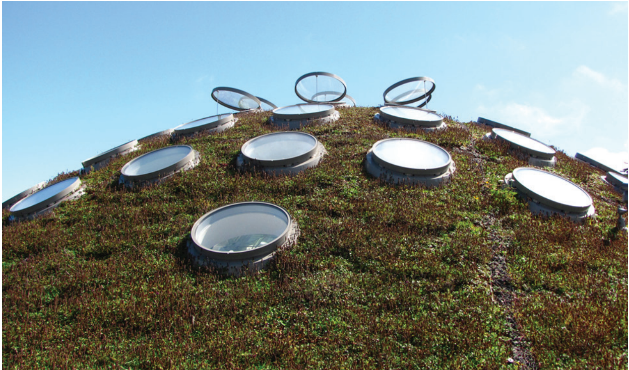
The roof of the California Academy of Sciences in San Francisco (Image: Orana Sandri, 2009)
