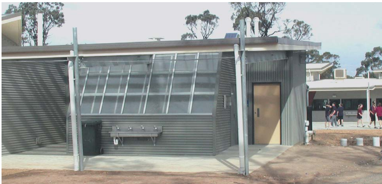
Figure 1 The urine-separating dry composting toilet block
