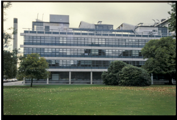
Figure 3 The south-west elevation of the teaching block
