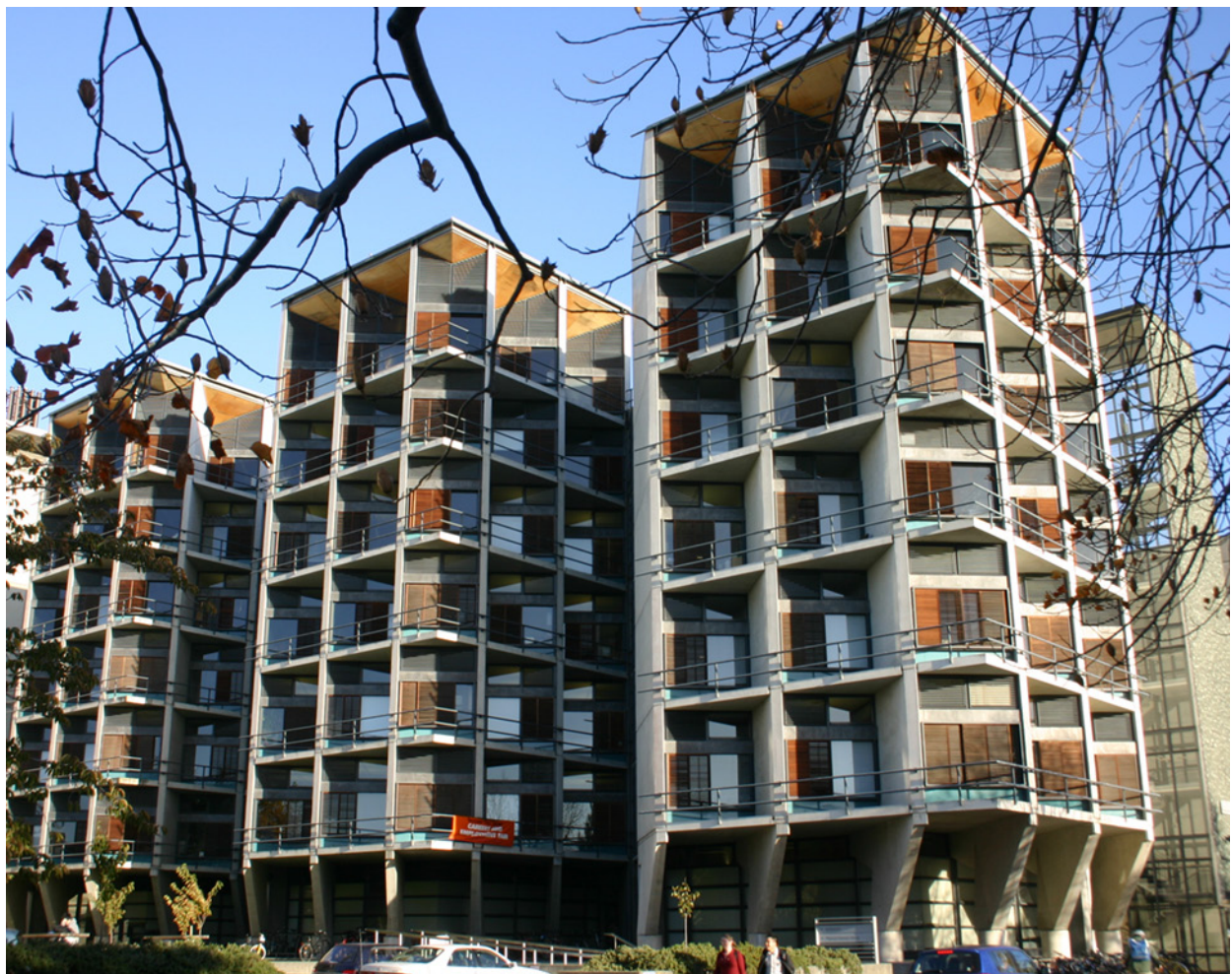
Figure 1 View from the north of the academic towers
