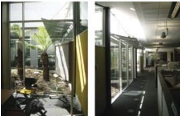
Figure 4. External and internal views of light shelves for courtyard
