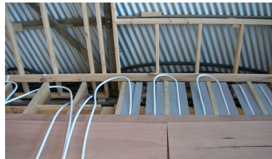
Figure 9. Second floor studio hydronic heating system
