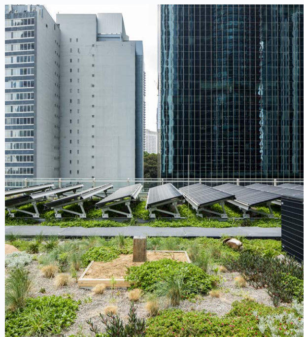
Figure 5. The integrated green roof — a mixture of natives and exotic plants aims to support biodiversity within the urban environment (Image: Brett Boardman).
