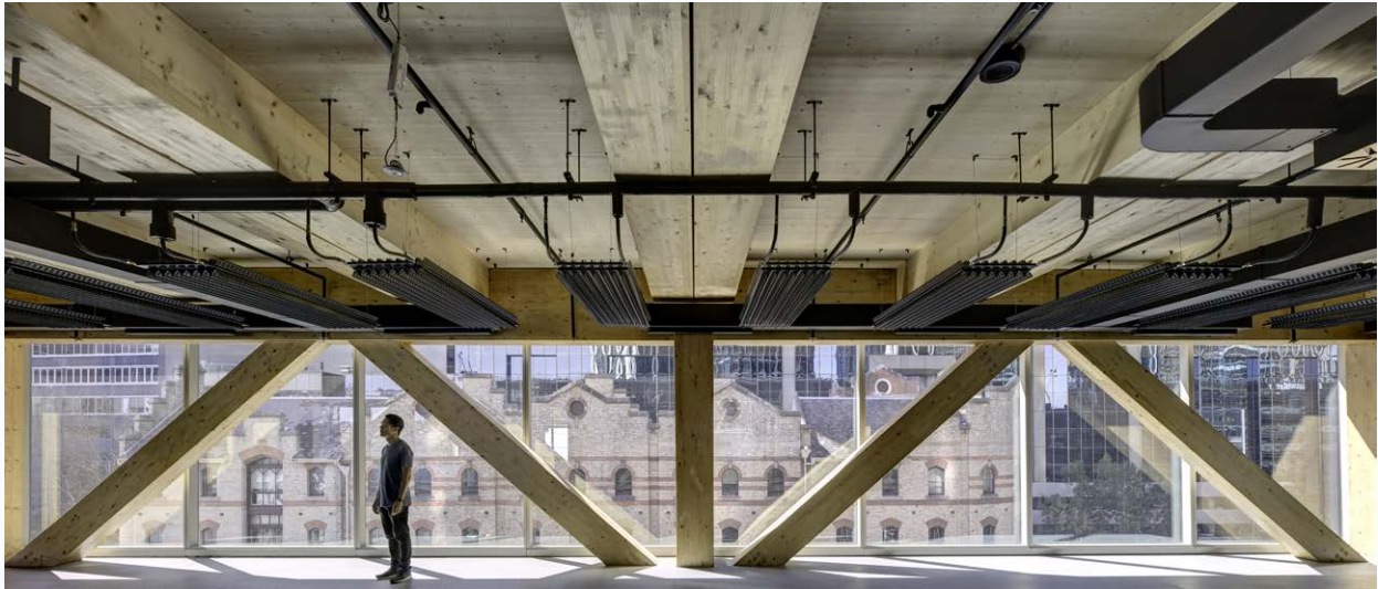
Figure 11. View of a typical commercial interior — exposing the services maximises the presence of the timber structure to improve the biophilic benefit to the workplace (Image: Brett Boardman).
