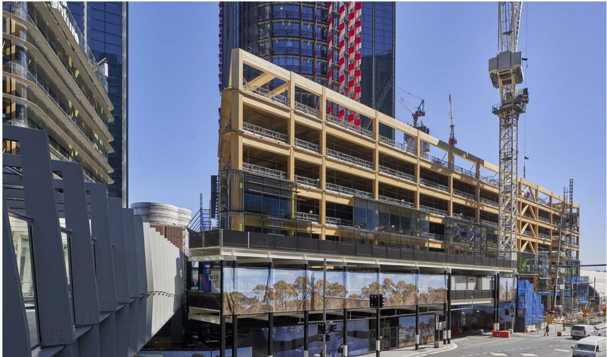
Figure 6. Daramu House under construction — building without scaffolding exposes the process of construction to the public (Image: Michael Nicholson).
