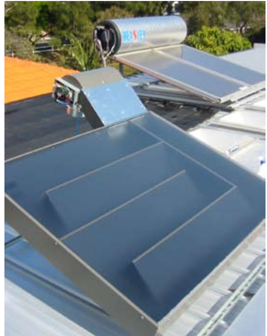
Figure 7. 'Sun Lizard' Solar Air Heater
