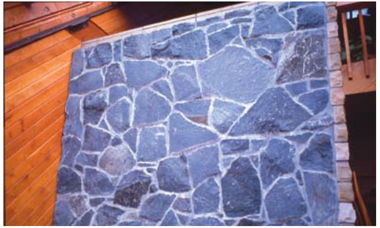
Fig. 2 A feature stone wall facing a north facing glass house is used in this house as the thermal mass
