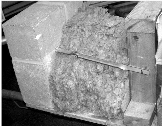
Figure 2. BedZed – detail of insulation of exterior walls (photograph by Nicholas Low of model by architect Bill Dunster)
