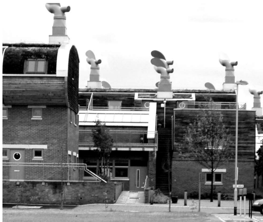
Figure 3. BedZed, showing the ventilation system
