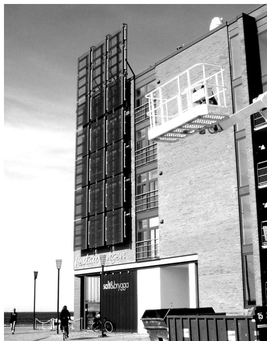
Figure 5. The Västra Hamnen development in Malmö. High efficiency solar collectors on the walls of an apartment block.
