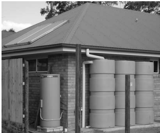
Figure 5. Rainwater tank and solar hot water system at Sanctuary Pocket, Forest Lake
