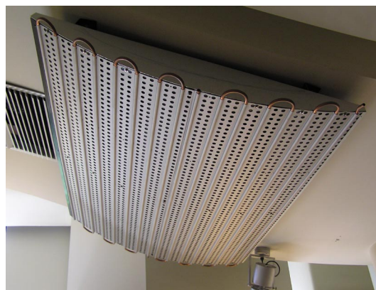
Figure 10. Chilled ceiling prototype
