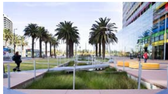
Figure 12. NAB Forecourt wetlands The chain link handrails were required to be retrofitted to increase pedestrian safety (Source: EDAW)
