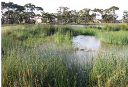
Figure 2. Wetland with permanent pool, Cairnlea Estate, Melbourne (Source: EDAW)
