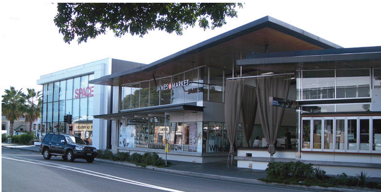
The slightly pitched roof over the central corridor expels hot air and assists passive cooling.
