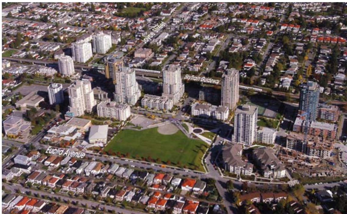
Figure 1. Joyce-Collingwood Station precinct in Vancouver
