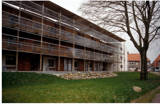
Garden block with screened verandahs for extra shelter
