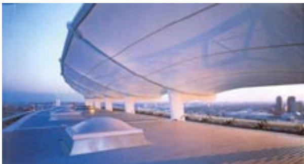
Figure 3: Seasonal sunlight occlusion for skylights
