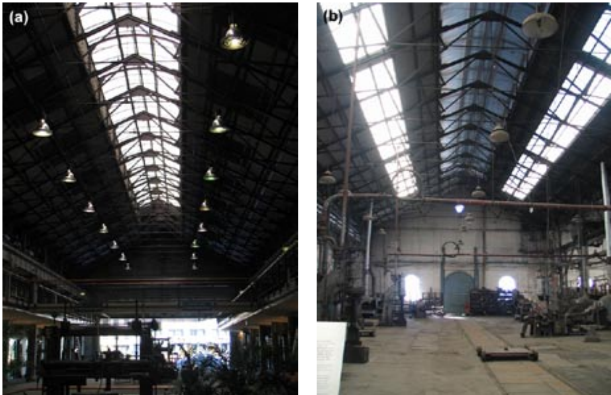
Figure 12: Identical adjacent buildings with different skylight arrangements (photos taken at the same time)
