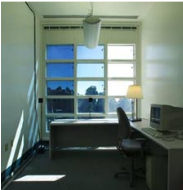
Figure 6: Demonstration of electrochromic windows 3
