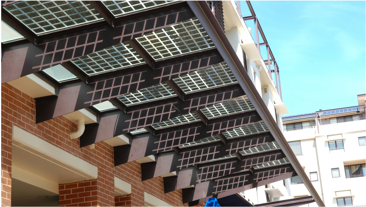
Figure 1 – Building-integrated photovoltaic application in Kogarah, NSW
