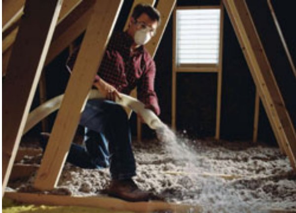
Blow-in insulation (Image: iStockphoto © Don Nichols 2009)
