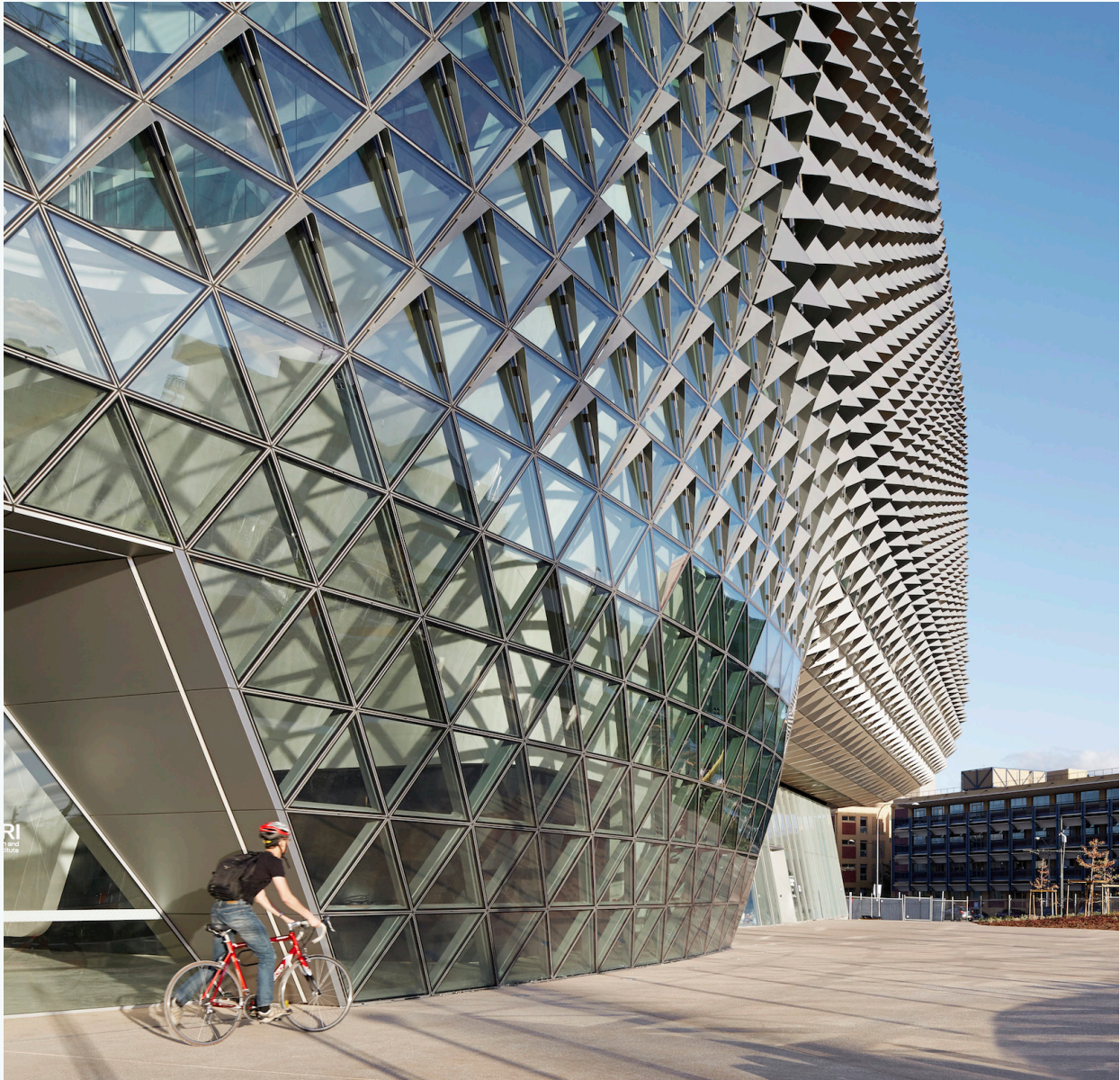
Figure 3. SAHMRI completed facade showing hood geometry (Photo: Peter Clarke)
