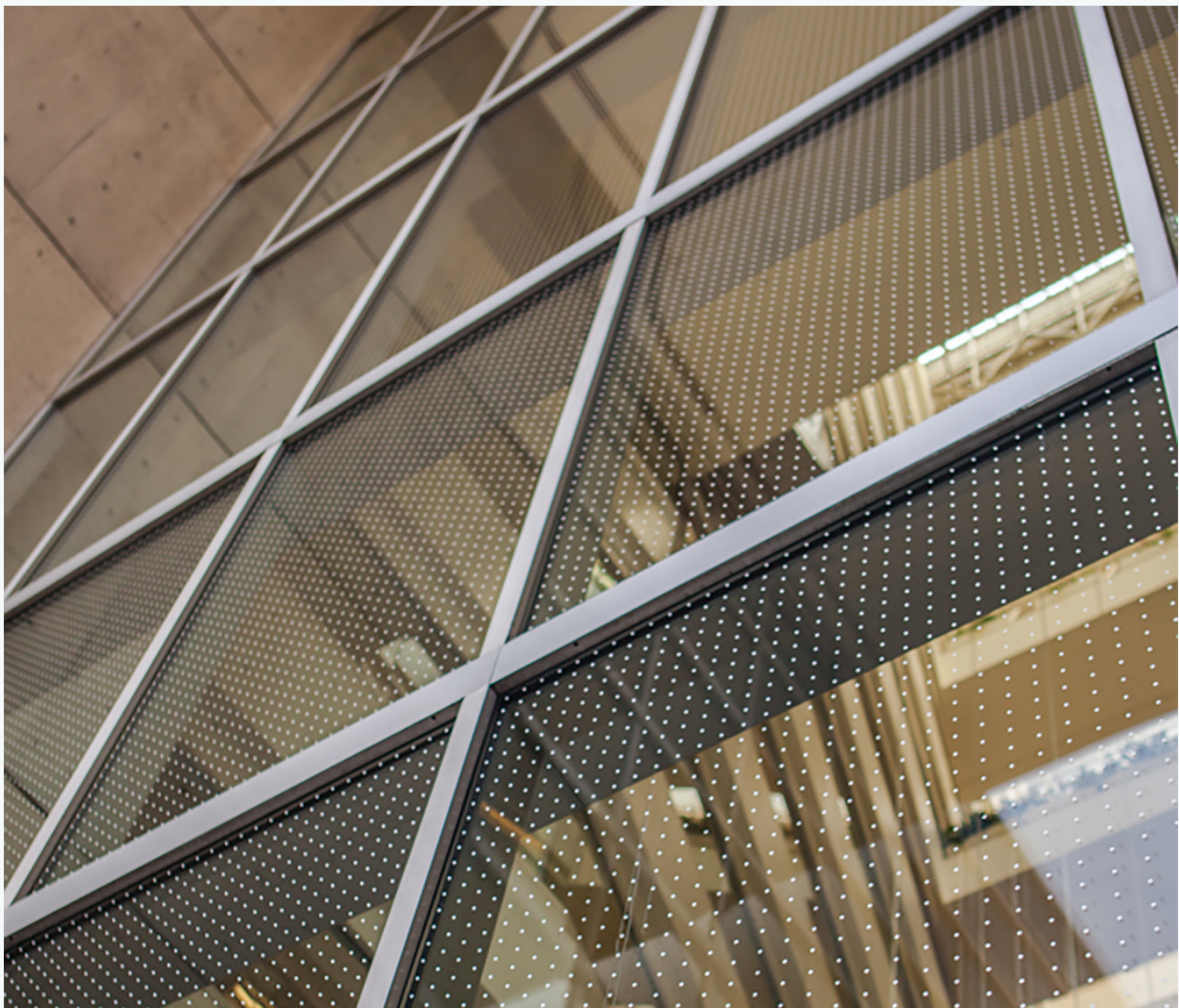
Figure 5. Dot markers applied to the exterior of the glass, visible to birds but unobtrusive to the building occupants (Image: Feather Friendly, 2018, www.featherfriendly.com ).
