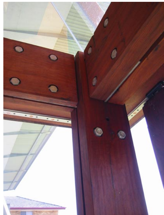
Figure 6. Connection detail – Harbour House
