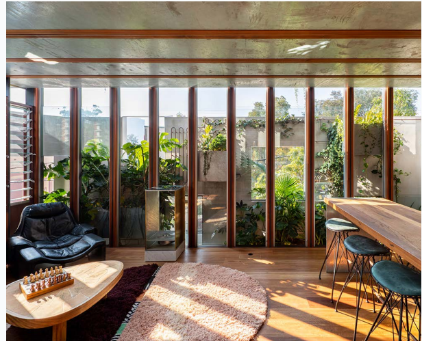
Figure 12. 600mm cavity between facade layers (Image: Michael Lassman)
