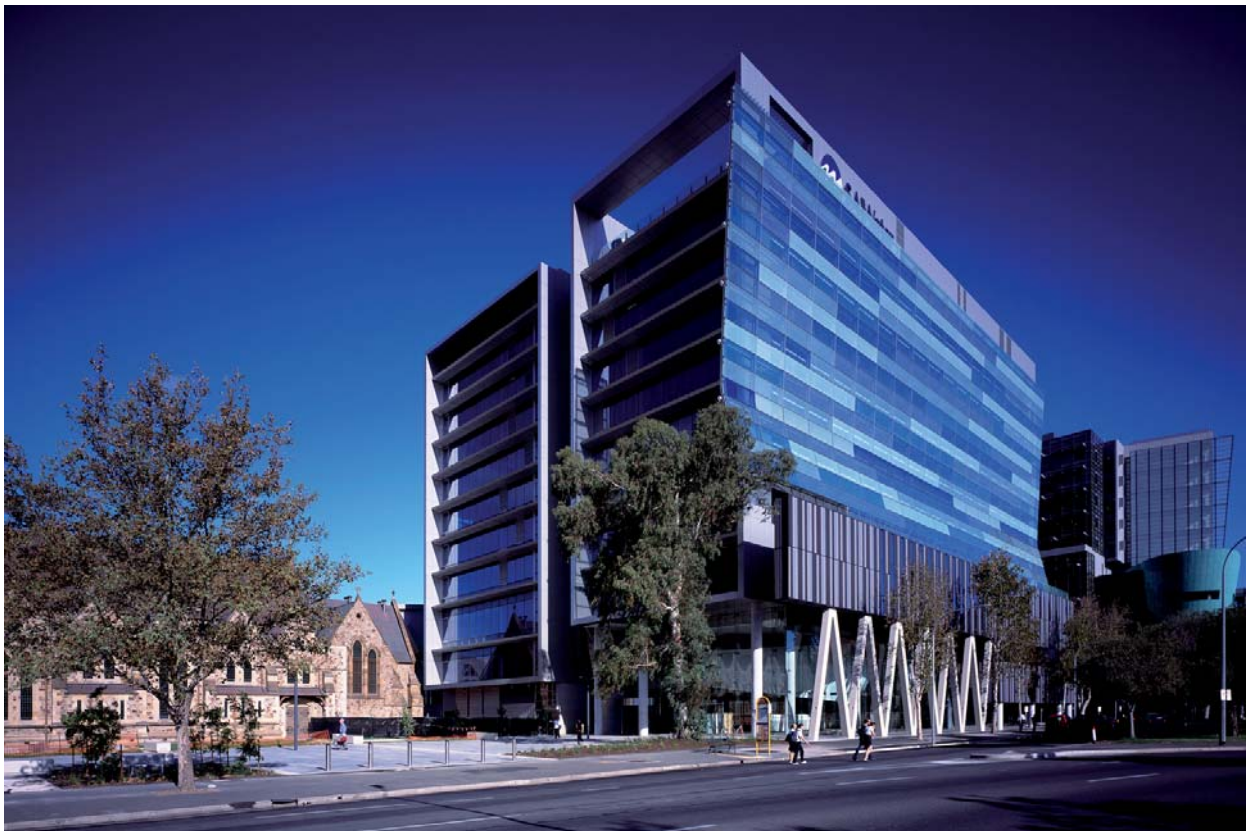
Figure 1: SA Water House, Adelaide
