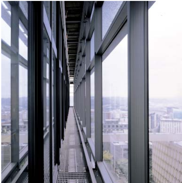
Maintenance platform between facades
