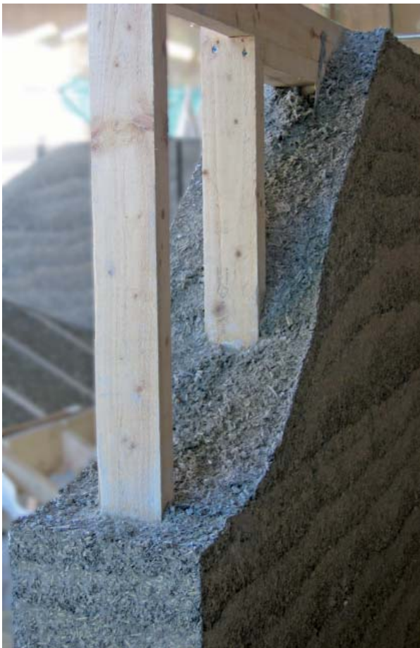
Figure 2: Hemp based products used for wall construction
