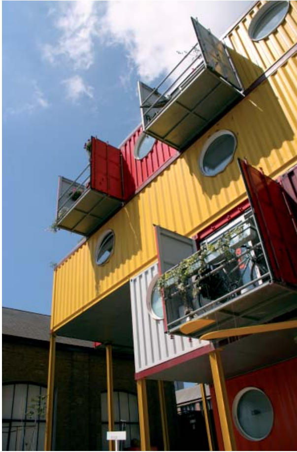
Figure 3: Shipping containers reused as accommodation
