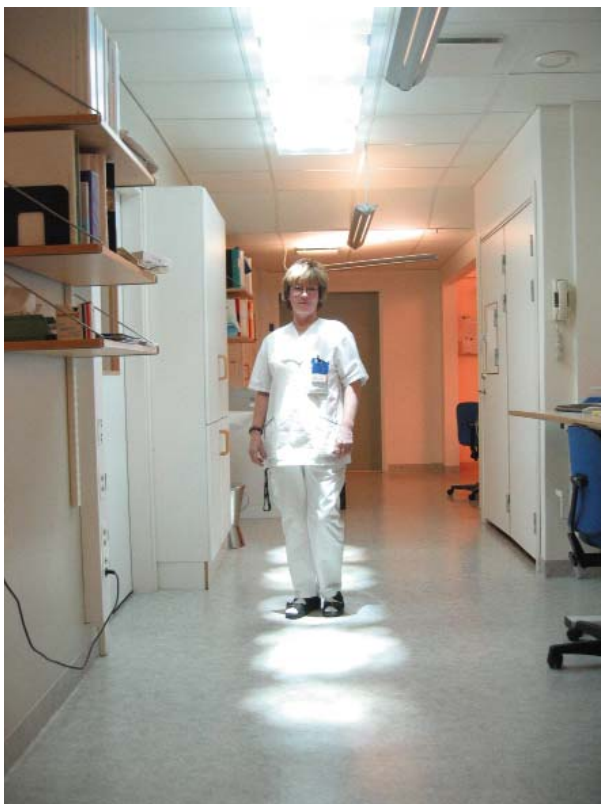
Interior light by optic fibre transmitted daylight
