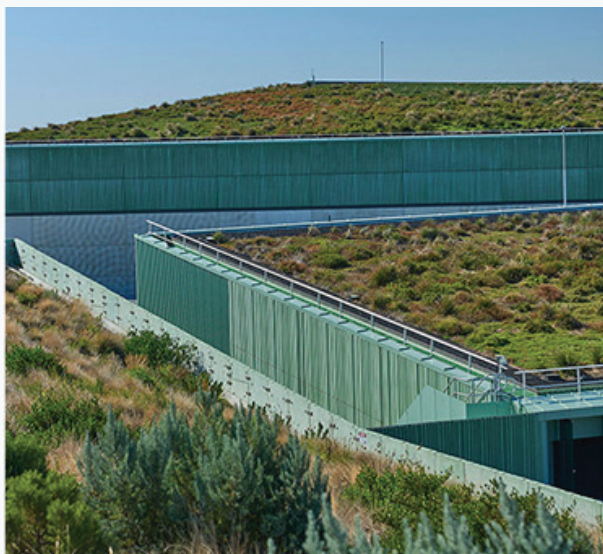
Figure 2. Victorian Desalination Project green roof, Wonthaggi, by ARM Architecture and peckvonhartel with ASPECT Studios. The green roof was designed to ameliorate the visual impacts of the development. (Photo: Aquasure)
