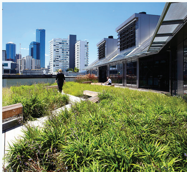
Figure 3. Kangan Automotive Centre of Excellence, Melbourne Docklands, by Gray Puksand with ASPECT Studios. This green roof reduces storm water run-off and provides amenity for building users. (Image: Andrew Lloyd)
