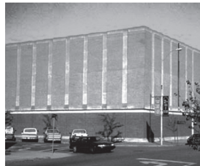
Existing building – shown before living walls are added
